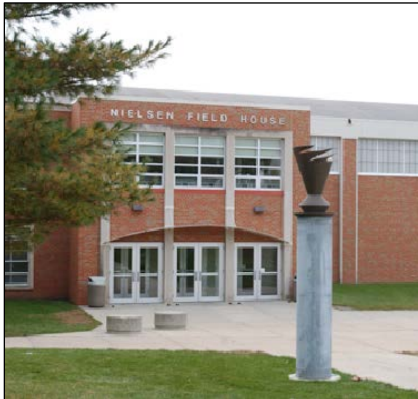
University of Northern Iowa's Nielsen Field House, north entrance, looking south
