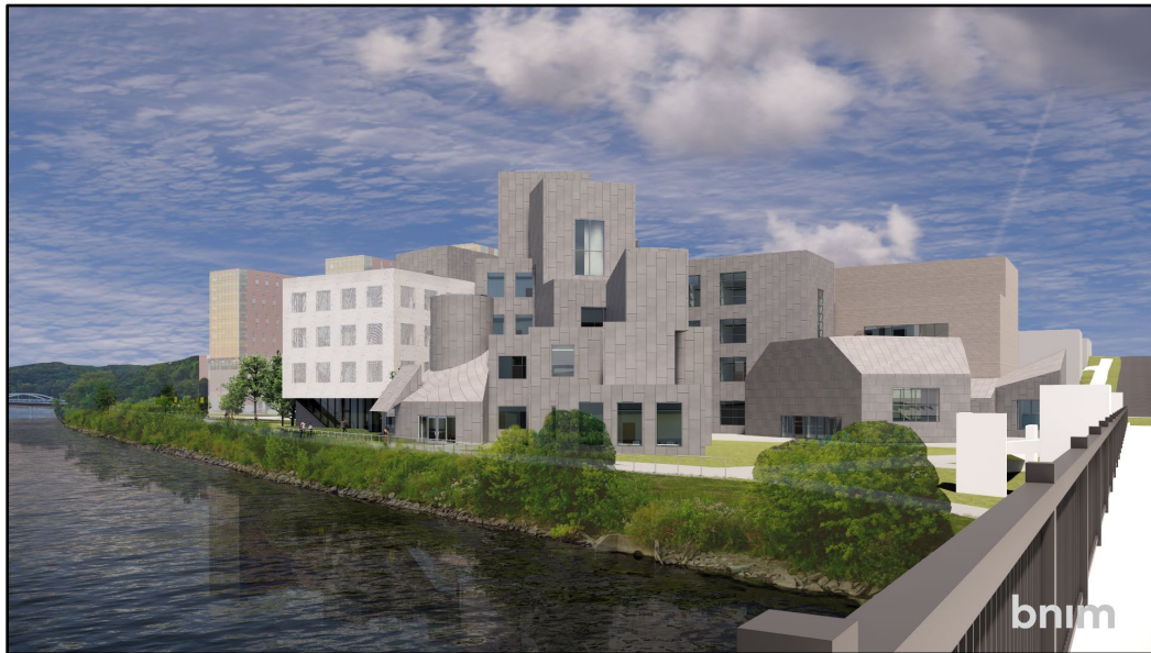
View from pedestrian bridge, looking northeast
