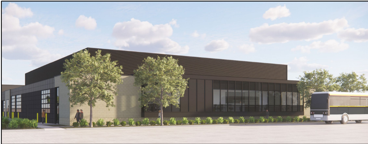
North of the new addition, looking southwest
