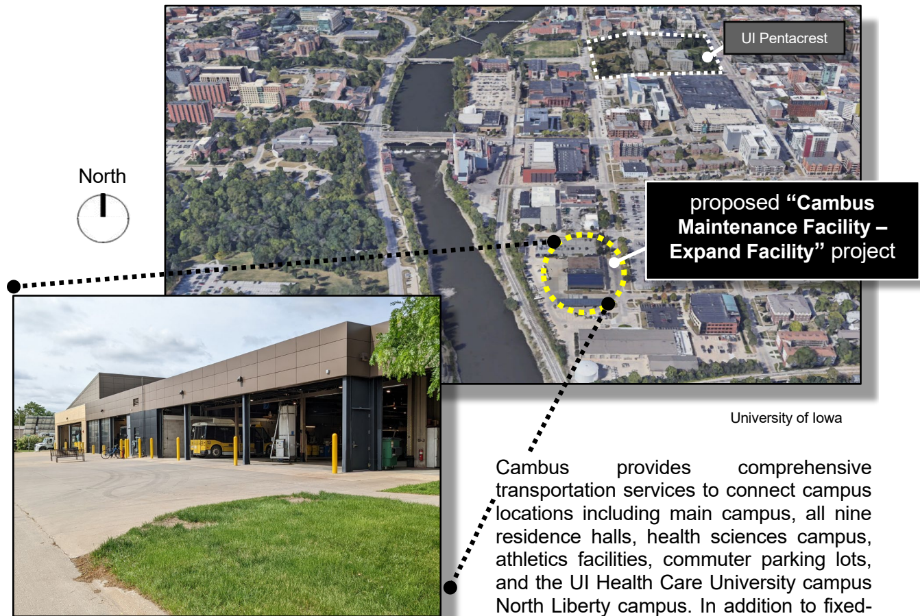
Existing Cambus Maintenance Facility, looking southwest
