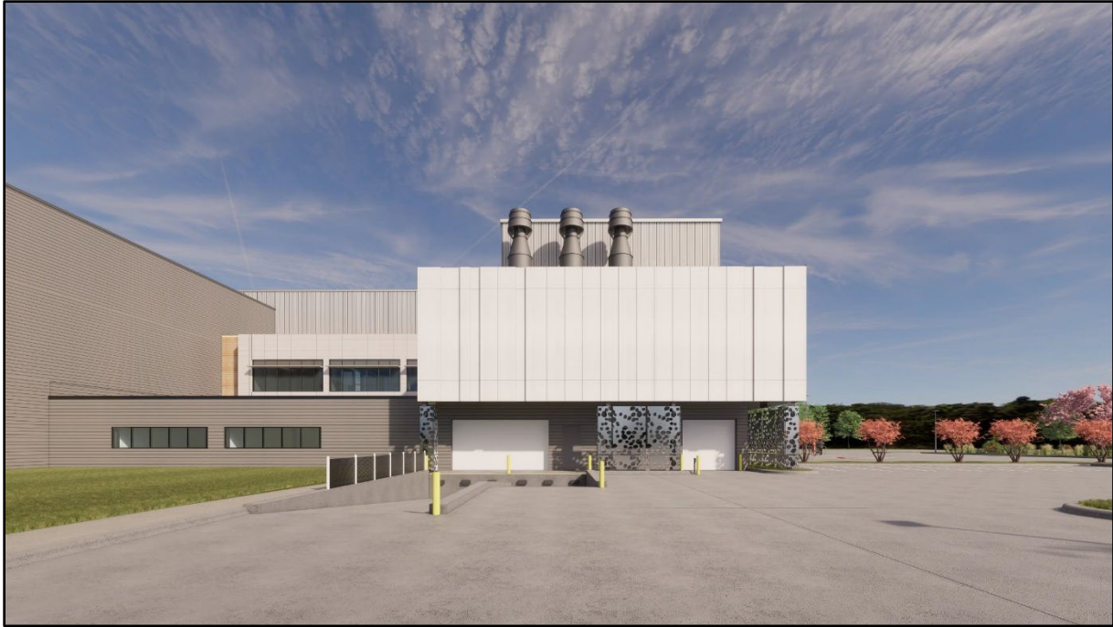
Loading Dock and Drive-Through Sample Drop Off, looking north
