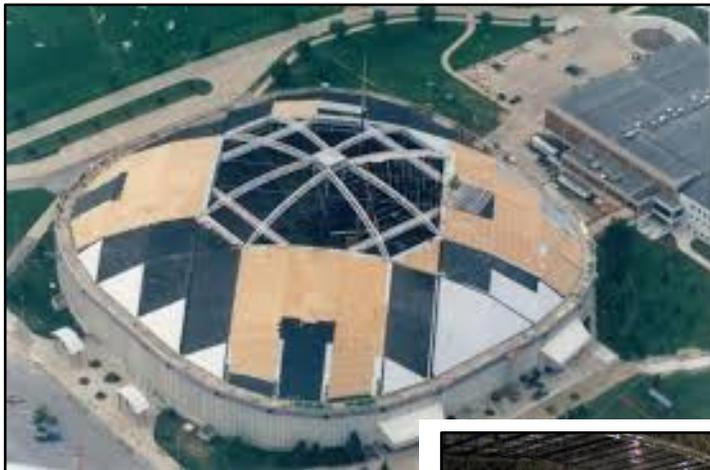
UNI-Dome's new 'hard' outer roof and the center portion's fabric roof, under construction in 1999
